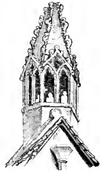
Chimney, Barford, Oxfordshire.
